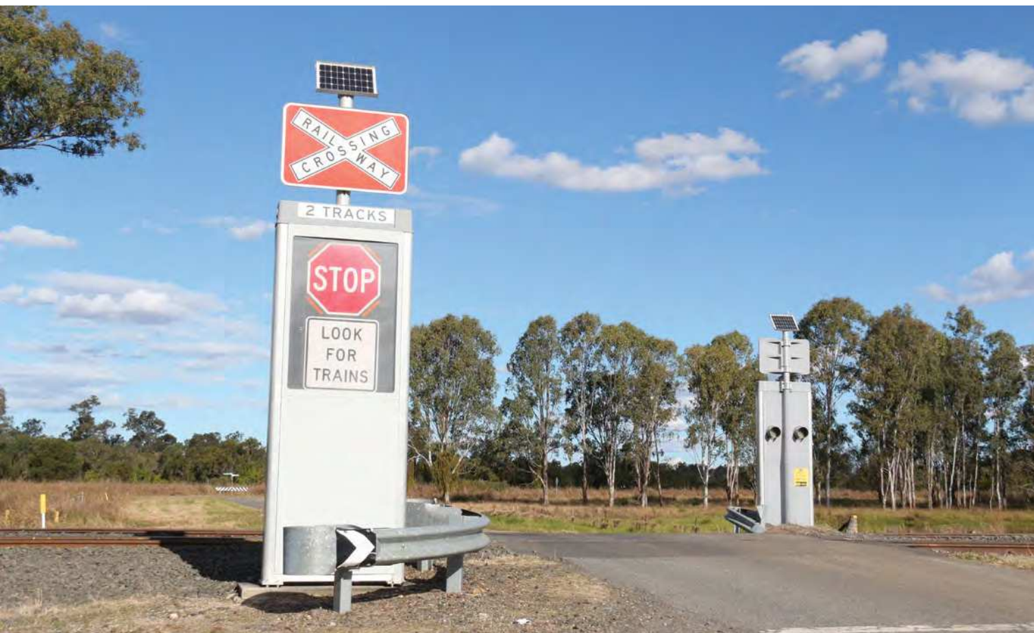
The level crossing at Lane Road, Lanefield, west of Rosewood, was equipped with flashing lights as part of a pilot project launched in 2015 involving Queensland Transport and Main Roads and Rail Safety Systems predecessor, Railnet Safety Systems. With the completion of the trial the crossing warning lights were de-activated and converted to stop signs as seen in this 18 June 2022 view. A similar installation was installed at the south western Queensland town of Thallon.
